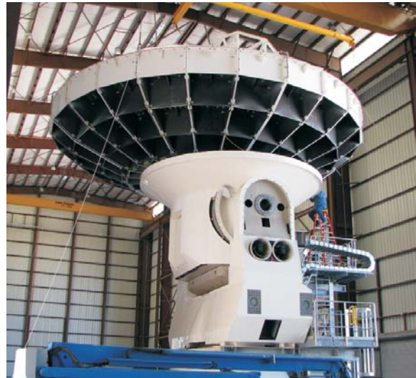
Figure 5. The pedestal for Vertex Antenna No. 3 and the backup structure have now been mated. VertexRSI antenna No 2, fully assembled, is in the Site Erection Facility.
