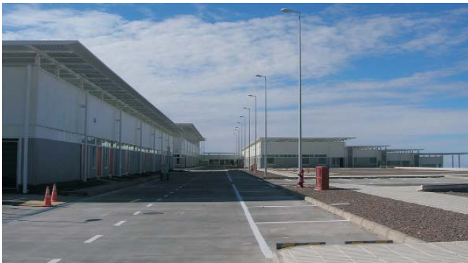
Figure 3. Construction on the OSF technical facility complex has been completed. The antenna assembly building (left) and technical building (right) are shown here.
